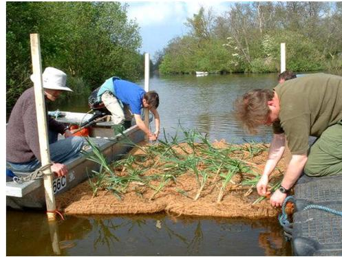
**Figure 1.** Installation of a coir pallet and planting of bulrush *Schoenoplectus lacustris* and reedmace *Typha latifolia*.
